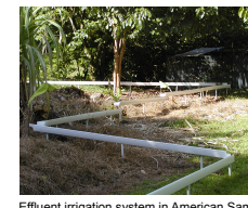
Effluent irrigation system in American Samoa
